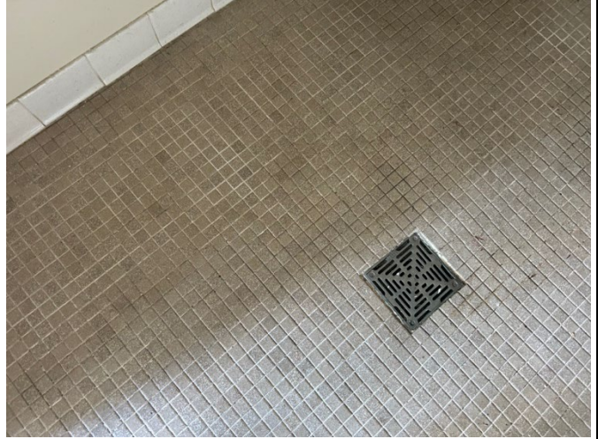
GROUT/MORTAR 1"X1" CERAMIC FLOOR TILE - OFFICE BATHROOMS
